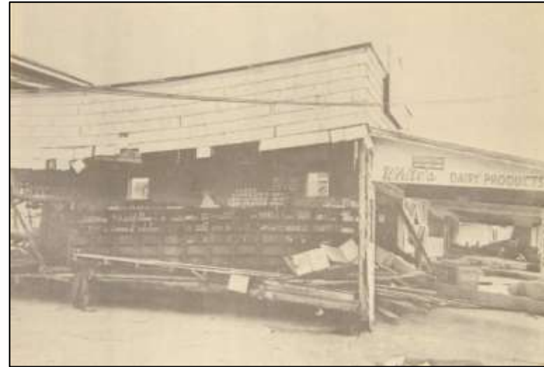
Hurricane Hazel (1954) – Typical Business Damage
